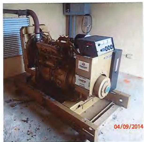
Figure 6: 200 KV E. Generator and ~280 gallons diesel ATS
