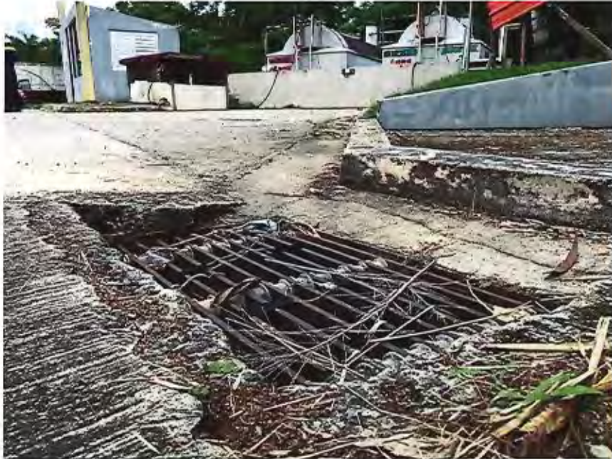
Figure 7: Storm Sewer near the Gas Station
