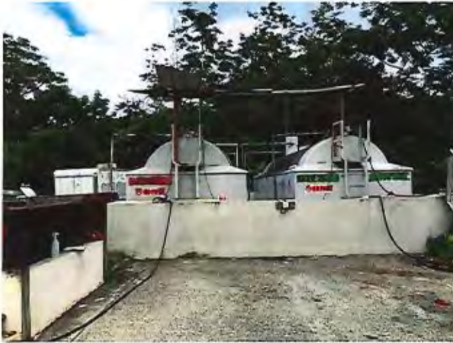
Figures 1 - 4: 10,000 Gallons diesel/gasoline aboveground store tanks
