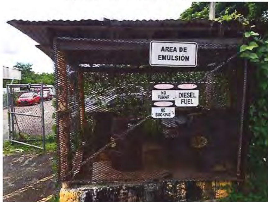
Figure 7: Emulsion oils storage site
