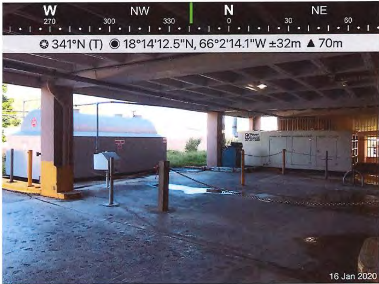
Figure 4: Caguas Municipal Government facility subject to SPCC Plan
