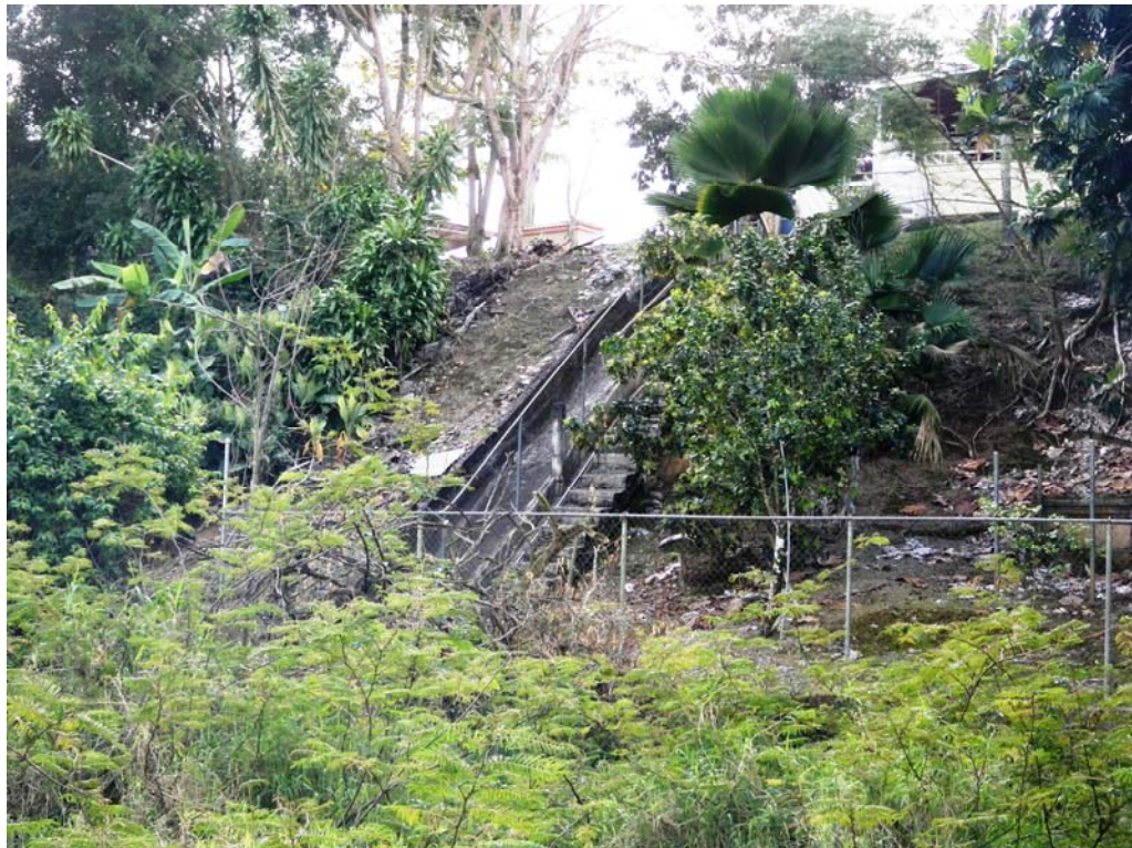
PHOTO 12: DRAINAGE CHANNEL FROM RESIDENTIAL DEVELOPMENT IN TO ISOLATED WETLAND OUT SIDE PROJECT'S LIMIT.
