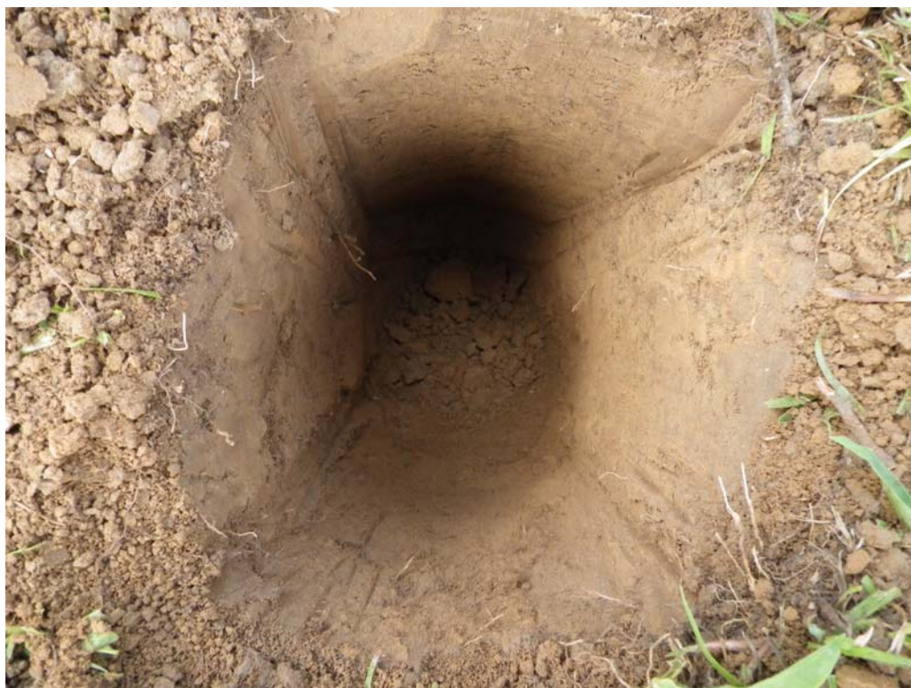
PHOTO 6: SOIL BORING AT SP-7.
